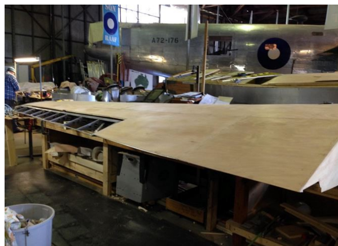
The port wing nearing completion – RAAF B-24 Liberator A72-176 can be seen in the background
