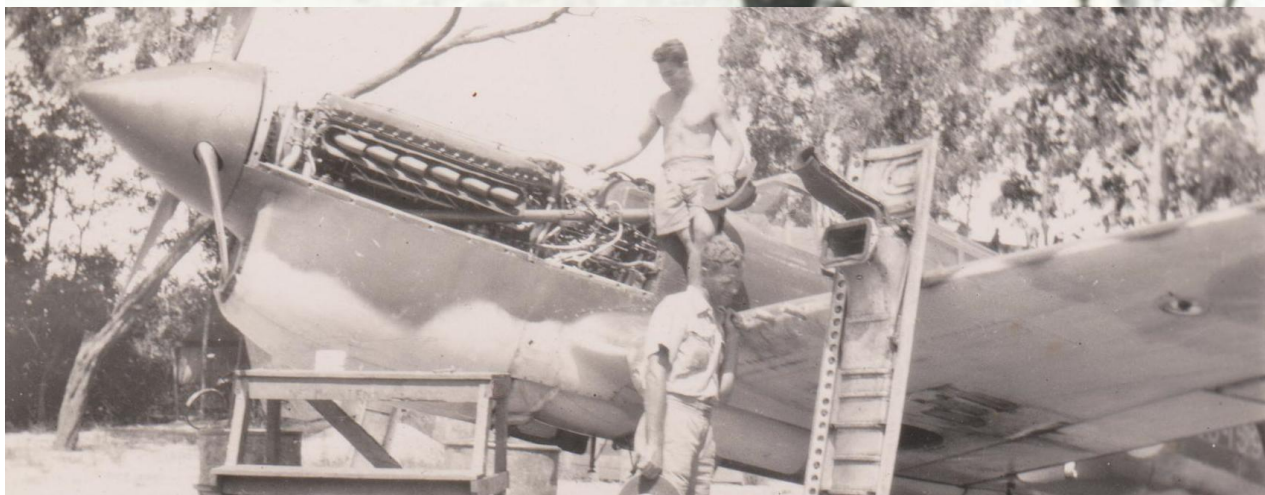
A29-159,....where did the Mossie go? Scalloping done to main plane boundary line.
