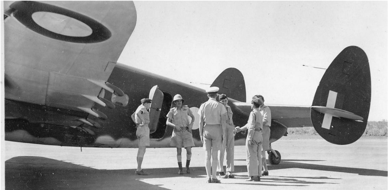
Other Hudsons, A16-98 as above, had been used by No 1 Communications Unit as a VIP Transport from January 1943 to December 1943 fitted with seven airline style seats. Pictured here transporting the then Chief of Air Staff (RAAF), AVM Jones to Batchelor NT. The Bath Tub had been covered over by streamlined sheeting.
